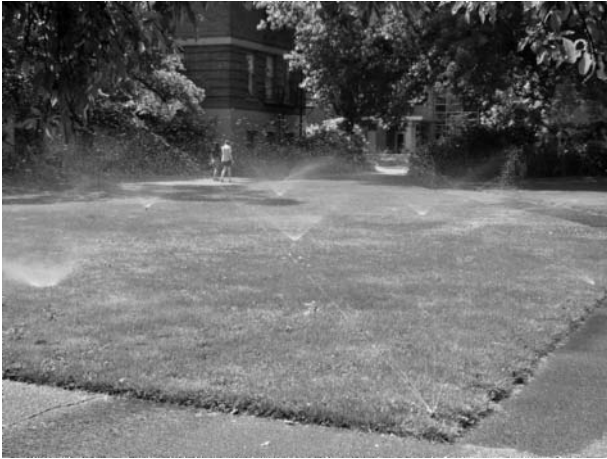
Figure 9-9 Mixing heads with different gpm (lpm) rates on the same zone makes it impossible to achieve uniform precipitation.
