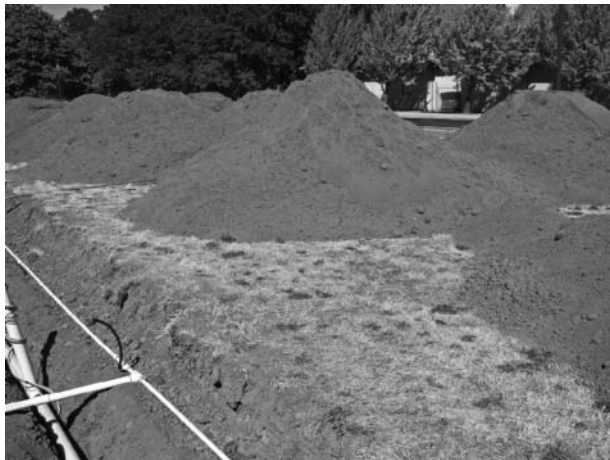
Figure 7-5 In this case, a loamy sand soil was placed over the original silty clay loam soil, resulting in nutritional and drainage issues.
