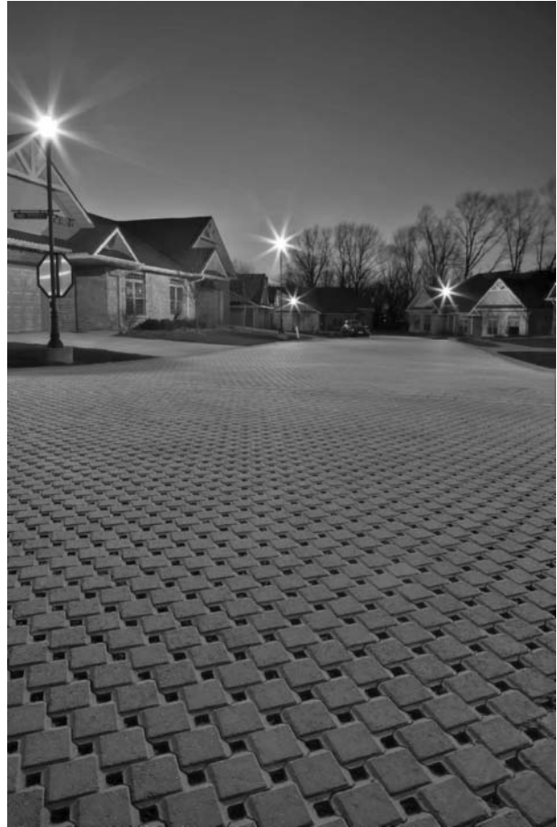
Figure 2-11 This development used permeable interlocking concrete pavers for the street and eliminated storm water runoff from that area. Courtesy of Unilock, Inc.
