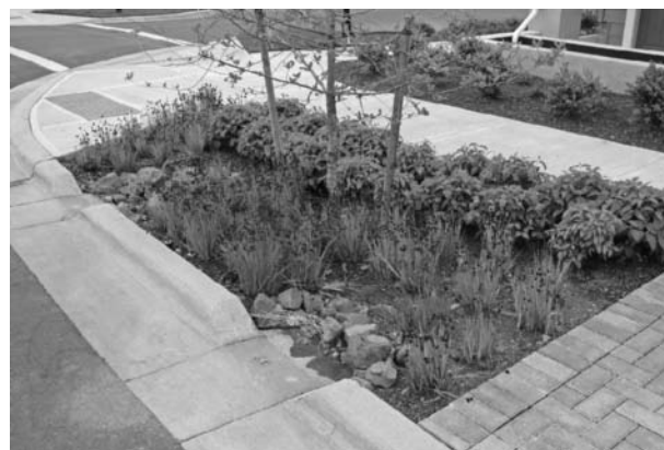
Figure 2-25 The small-scale rain garden shown here is an excellent way to collect water from hard surfaces, allowing it to filter through to the groundwater system.
