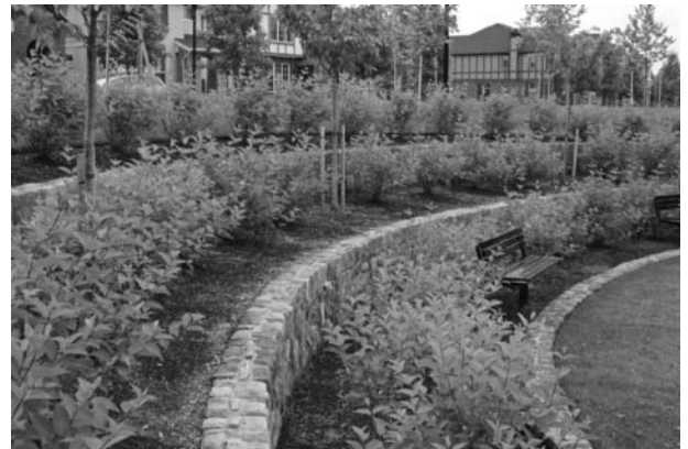
Figure 2-17 Short retaining walls were used to create level terraces for plantings in this design. The series of terraces gives the site an enclosed feeling and reduces noise from a nearby road.
